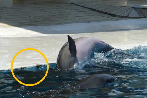
• Rust stains on the terracotta tiles near the bridge separating the main and smaller pools, indicating potential corrosion of the metal structural elements of the bridge and/or the barrier.
